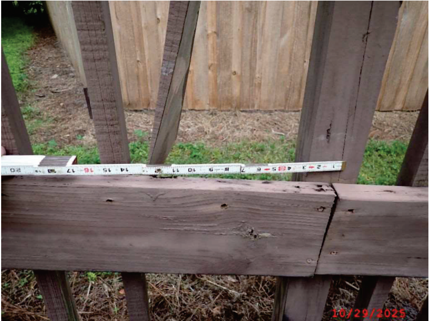
Photo 6: Element 332 Timber Bridge Railing
