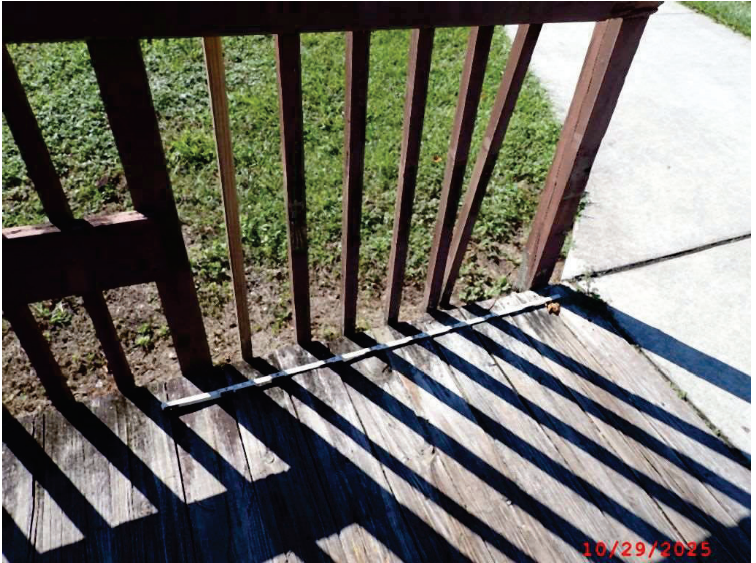
Photo 3: Element 332 Timber Bridge Railing
