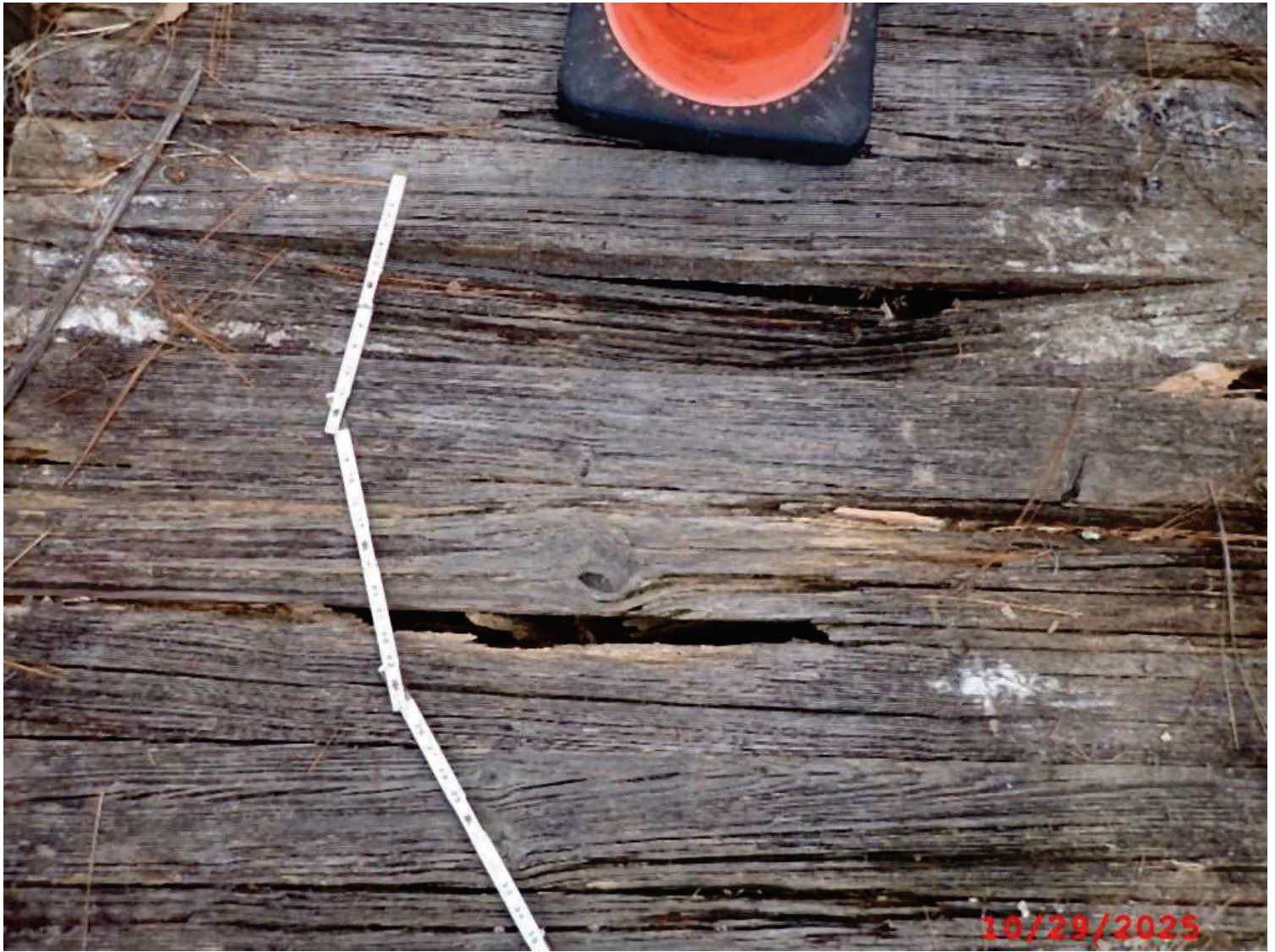
Photo 2: Element 31 Timber Deck
