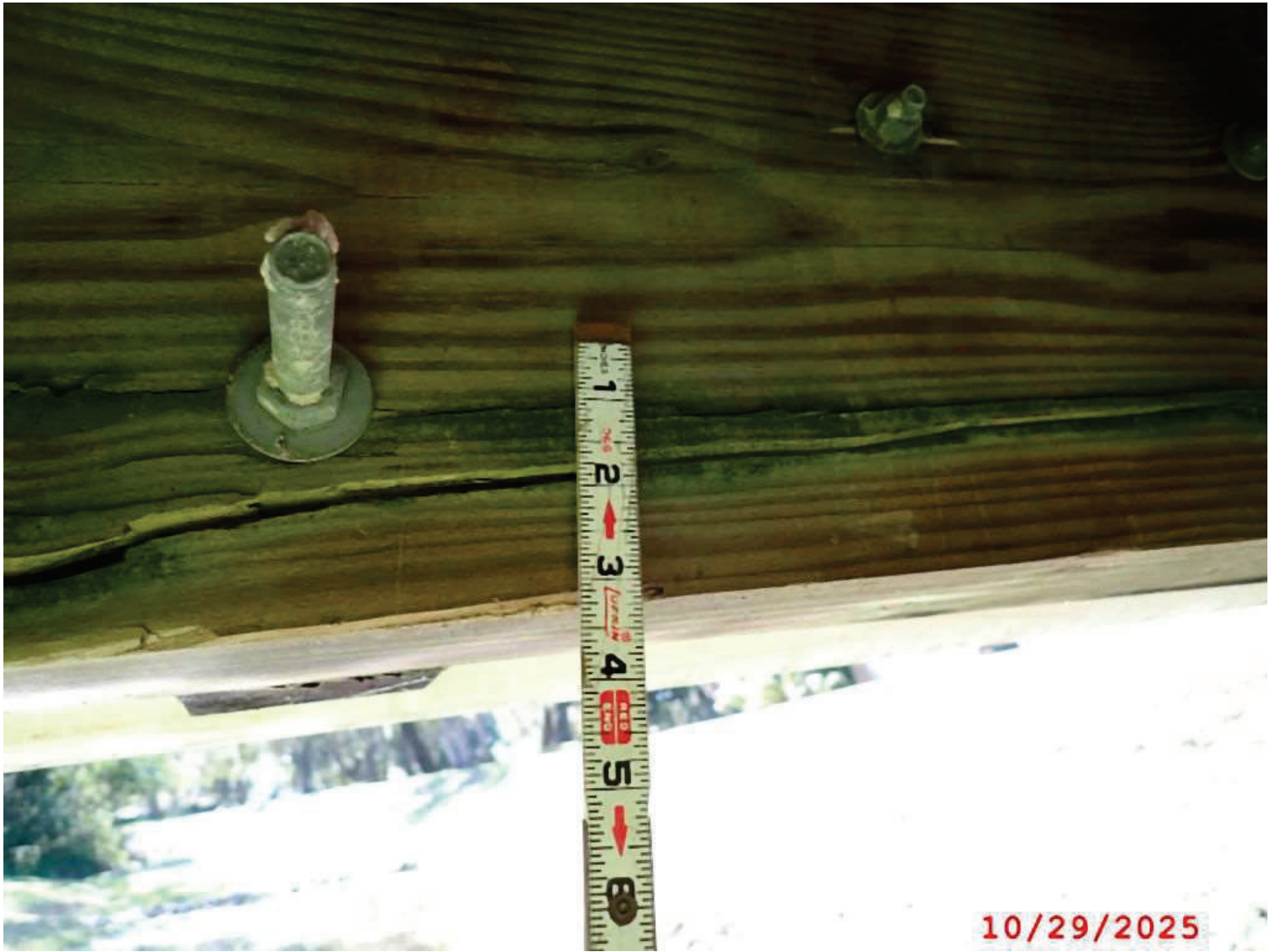
Photo 2: Element 111 Timber Open Girder
