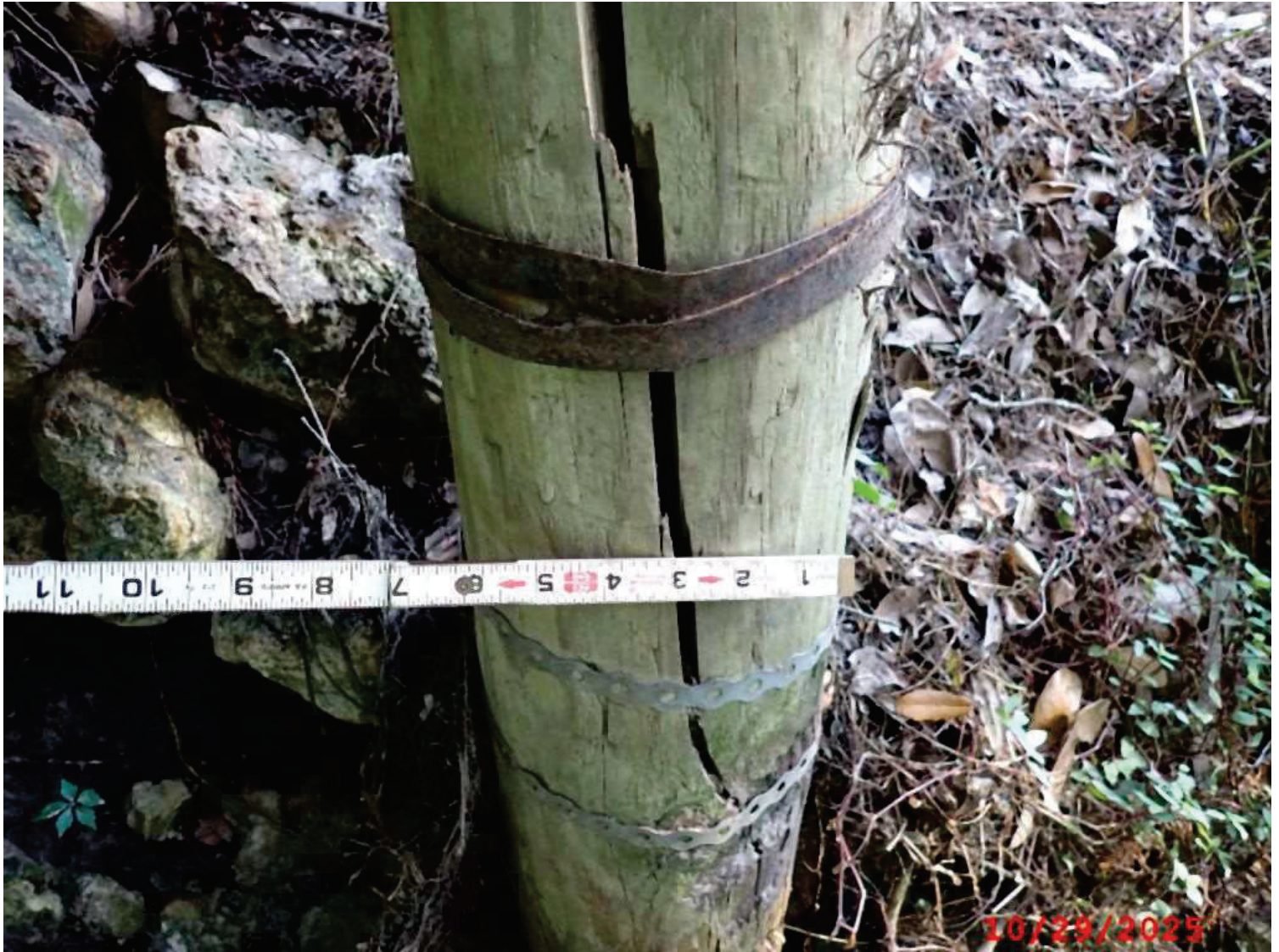
Photo 5: Element 228 Timber Pile
