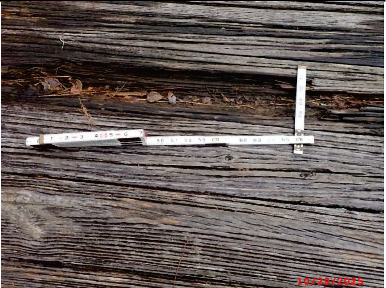
Photo 1: Element 31 Timber Deck
