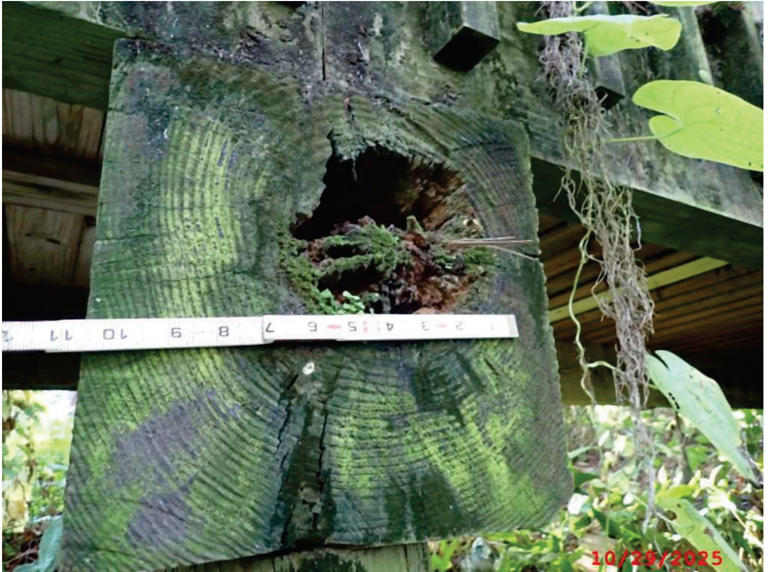
Photo 3: Element 235 Timber Pier Cap
