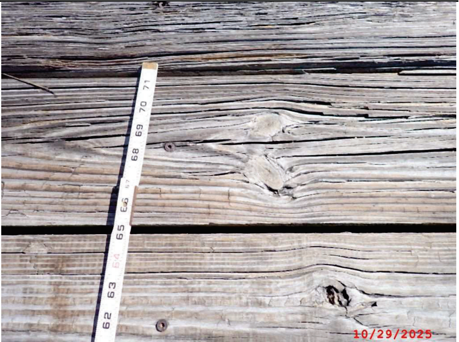
Photo 1: Element 31 Timber Deck
