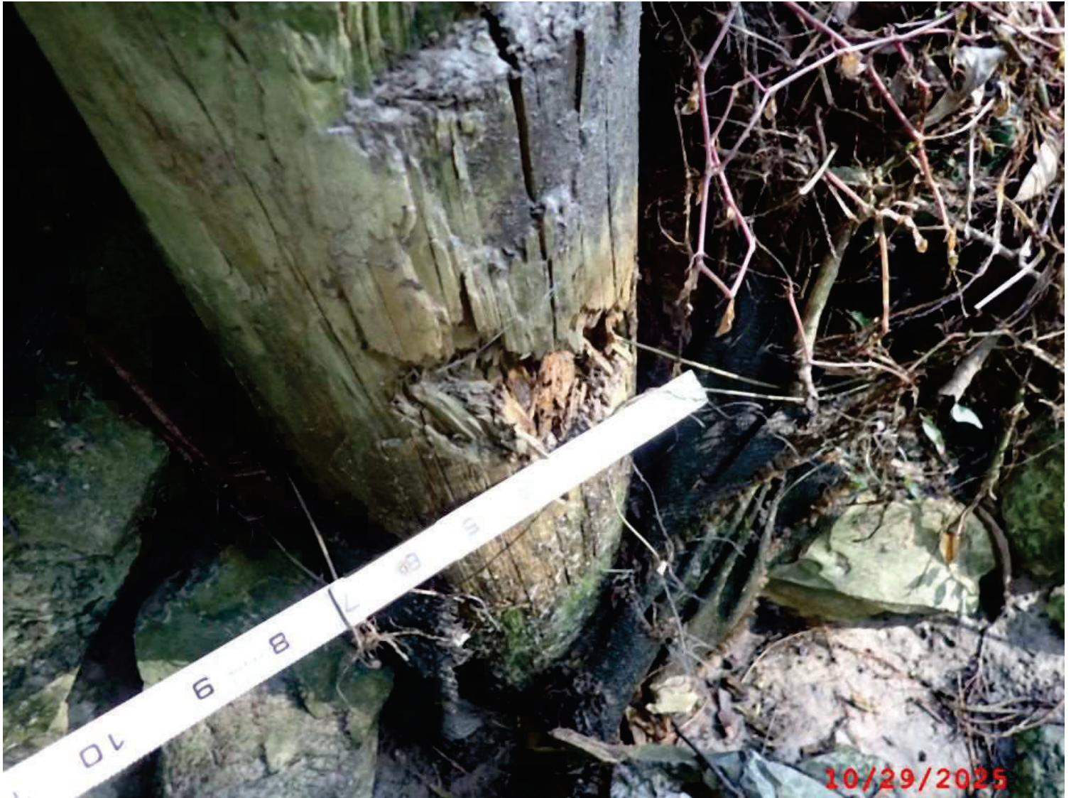
Photo 4: Element 228 Timber Pile
