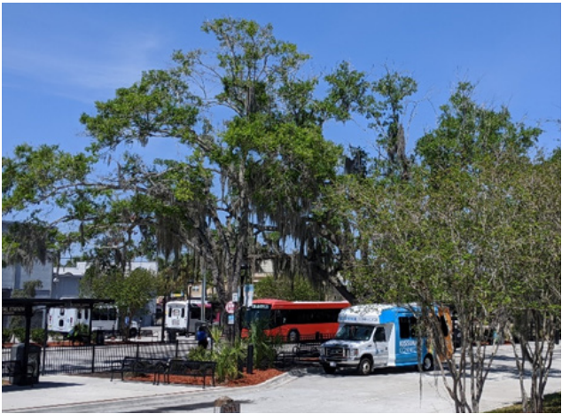
Figure 14.1 Kissimmee Intermodal Station
