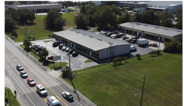
WAREHOUSE ON DYER BLVD
