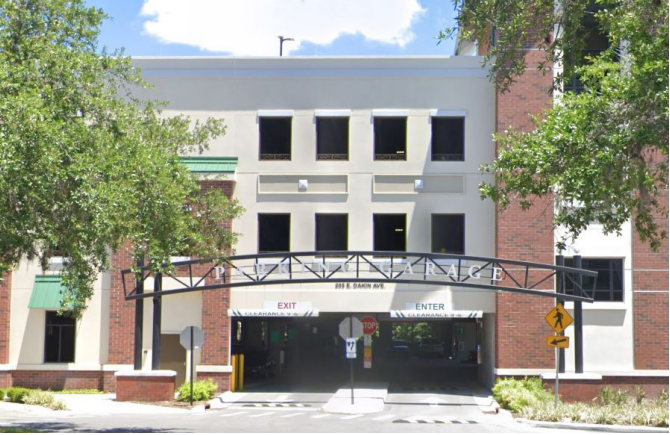
Figure 10.4 Intermodal Station Parking Garage
