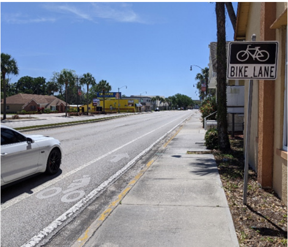
Figure 13.1 Bike Lane Signage and Conditions
