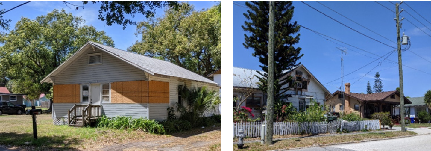
Figure 7.1 Examples of Deteriorating Housing
