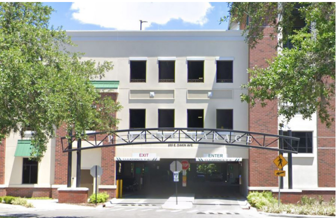
Figure 10.4 Intermodal Station Parking Garage
