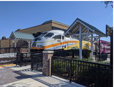
Figure 14.1 Kissimmee Intermodal Station
