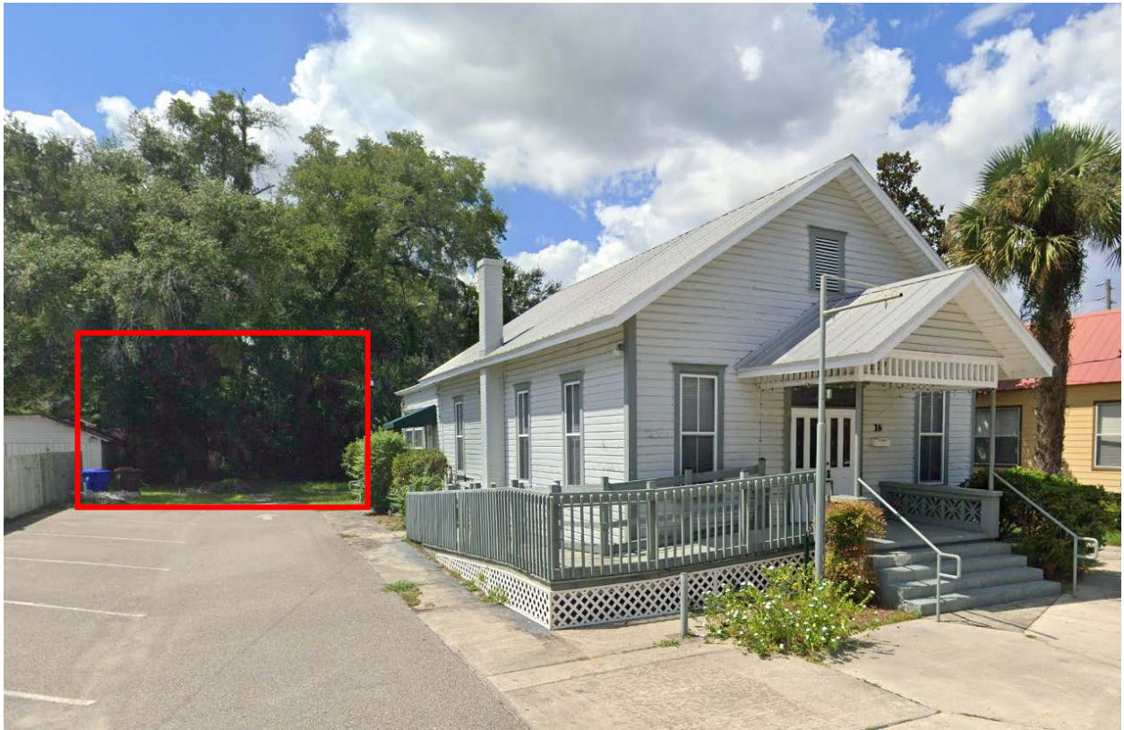
16 N. Orlando showing the shed location.
