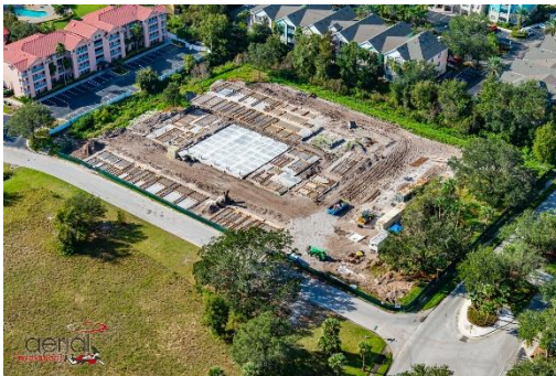
Fire Station 73 Site
