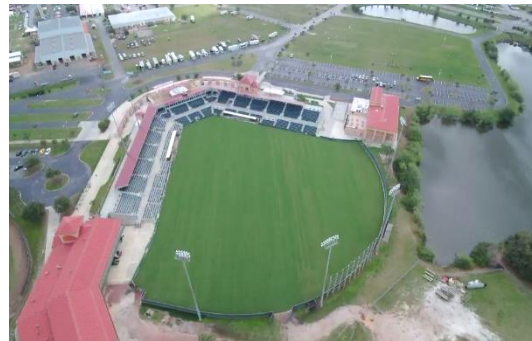
Osceola County Stadium Drainage
