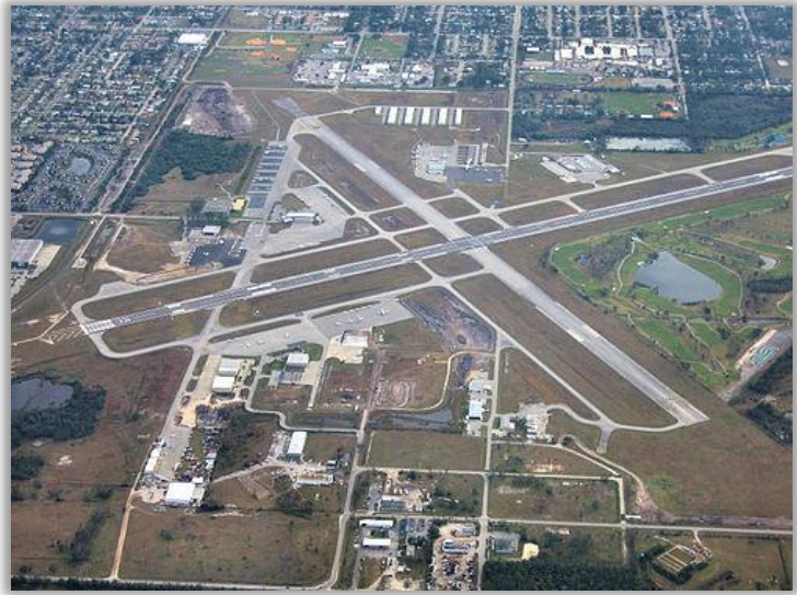
Figure 7 Kissimmee Gateway Airport
