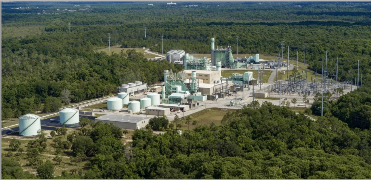
Figure 13 Cane Island Power Plant, Compliments of KUA
