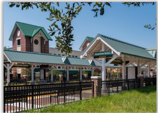
Kissimmee Intermodal Station, Courtesy of SunRail
