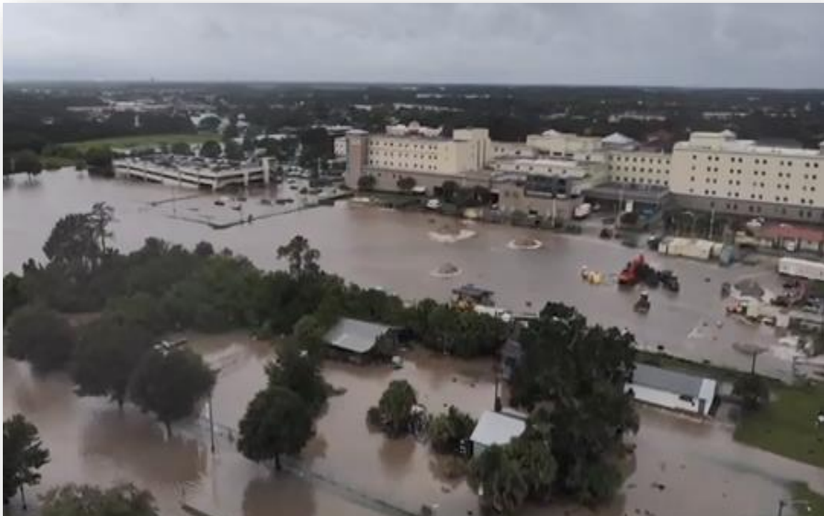
Flooding from Hurricane Ian September 29, 2022
