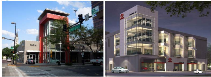
Figure 5-54: Auto Sales Facilities
