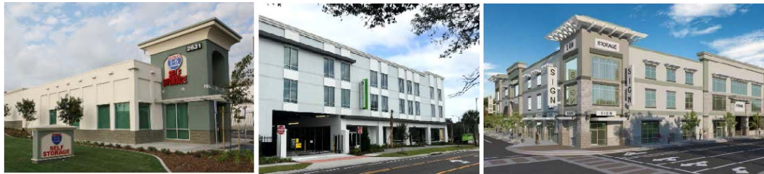
Figure 6-2: Examples of Self-Storage Facilities
