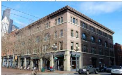
Taller ground to ceiling heights on the first floor provide flexibility for commercial use and a comfortable adjacent space for pedestrians
