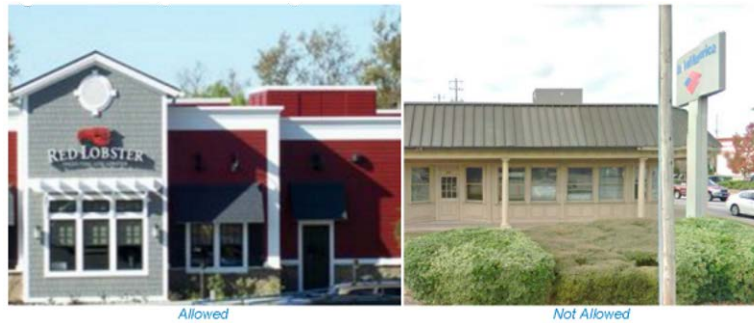
Figure 5-47: Rooftop Units Screening
