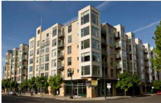
Taller floor-to-ceiling heights on the ground floor are more supportive of commercial uses
