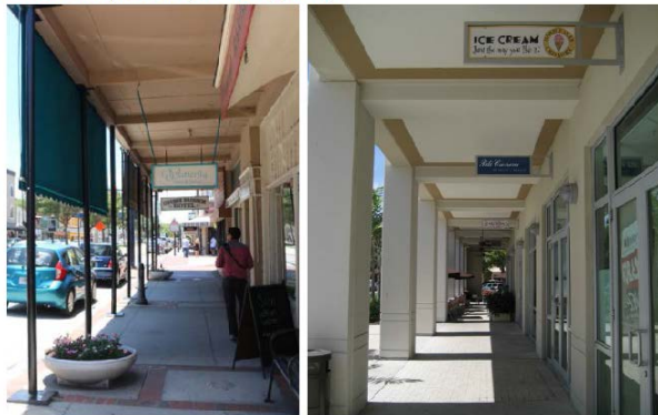
A gallery with slender metal columns (left) and masonry (right)
