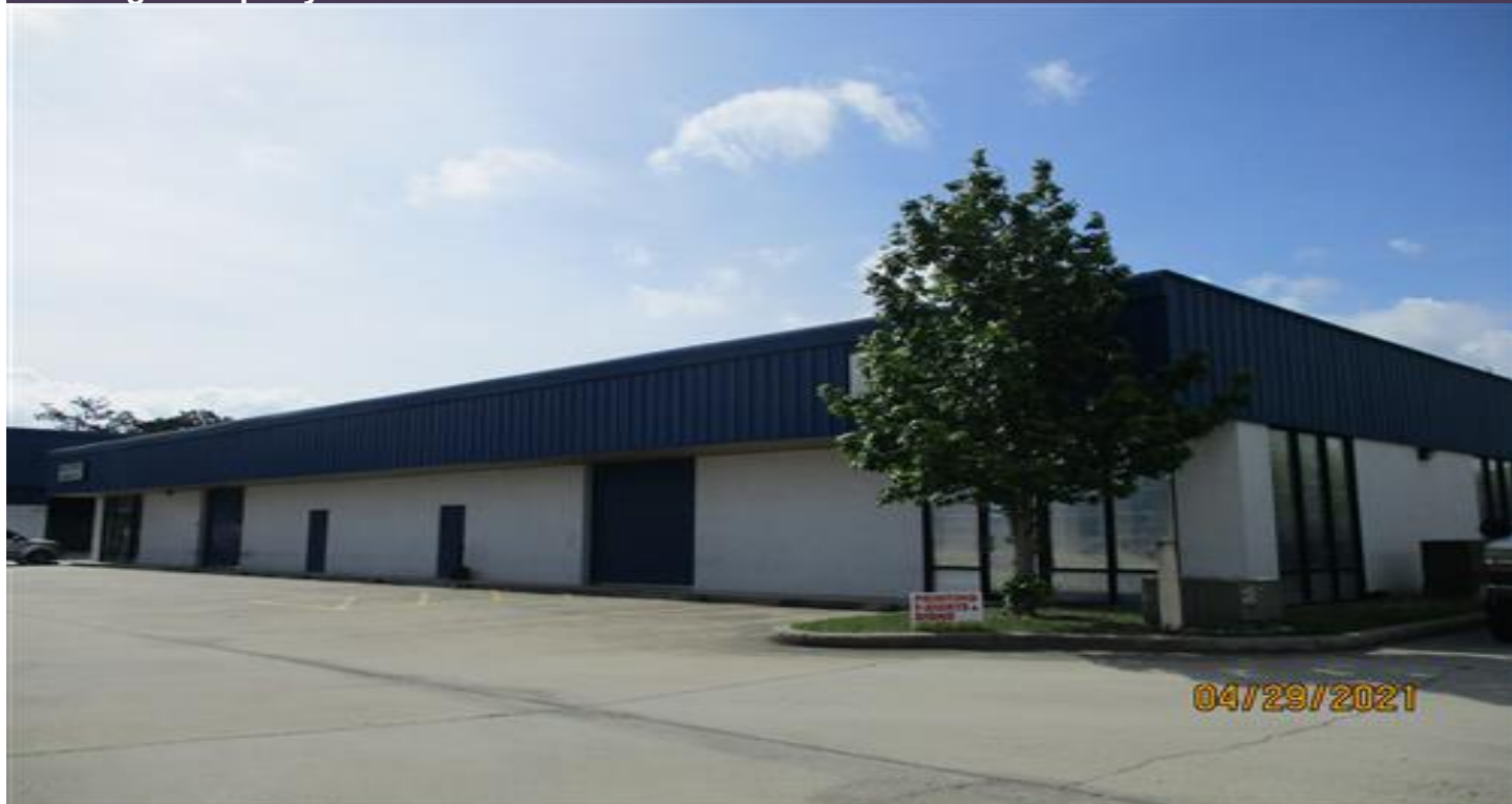
Building 2 Property Photo
