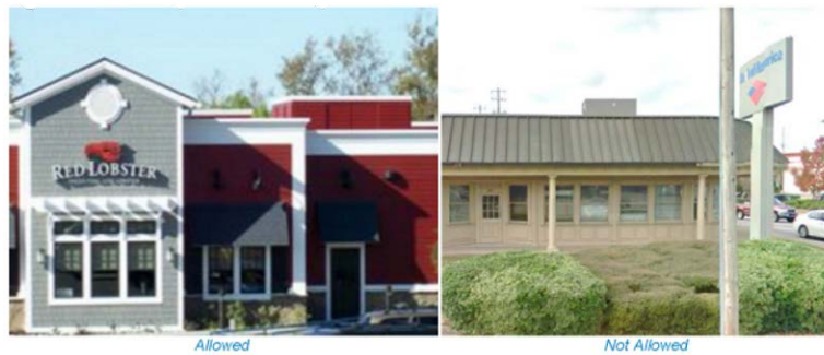
Figure 5-47: Rooftop Units Screening
