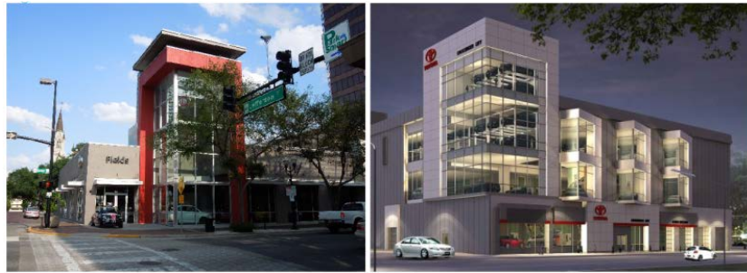
Figure 5-54: Auto Sales Facilities
