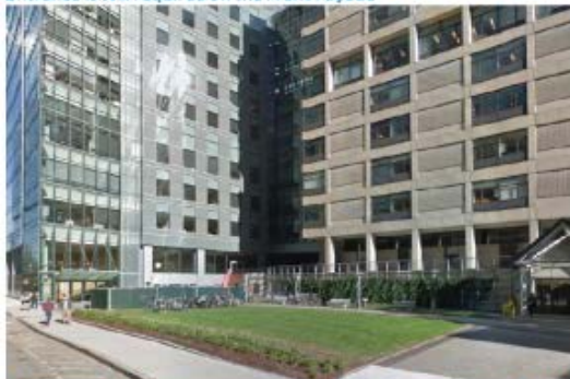
A portion of this building reaches the sidewalk while another portion is set behind a plaza
