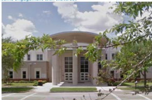
This school building fits its urban context by defining the street edge and providing an engaging pedestrian experience.
