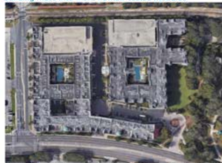
Aerial of mixed-use development. Buildings lining the street. Parking in the rear.
