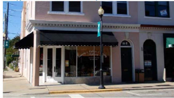
A shopfront with a chamfered corner entry
