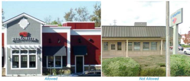
Figure 5-47: Rooftop Units Screening
