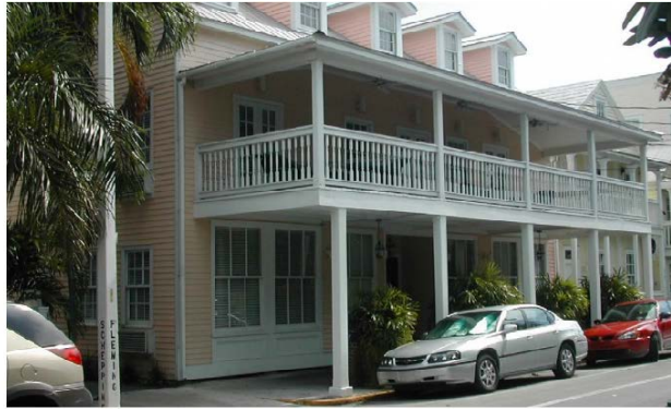
A two story wood framed gallery
