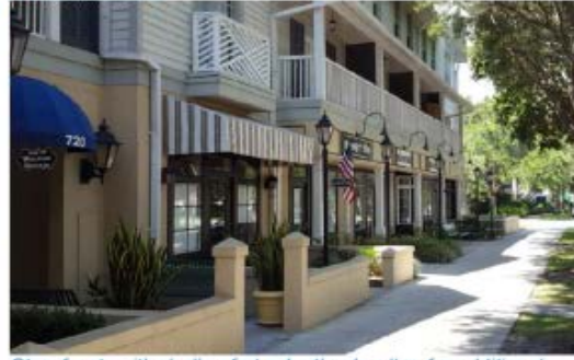
Storefronts with shallow front setbacks allow for additional landscaping and create a transition from the urban core to residential neighborhoods
