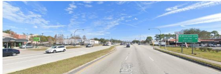
Looking east towards intersection with Michigan Ave. and Oak St.
