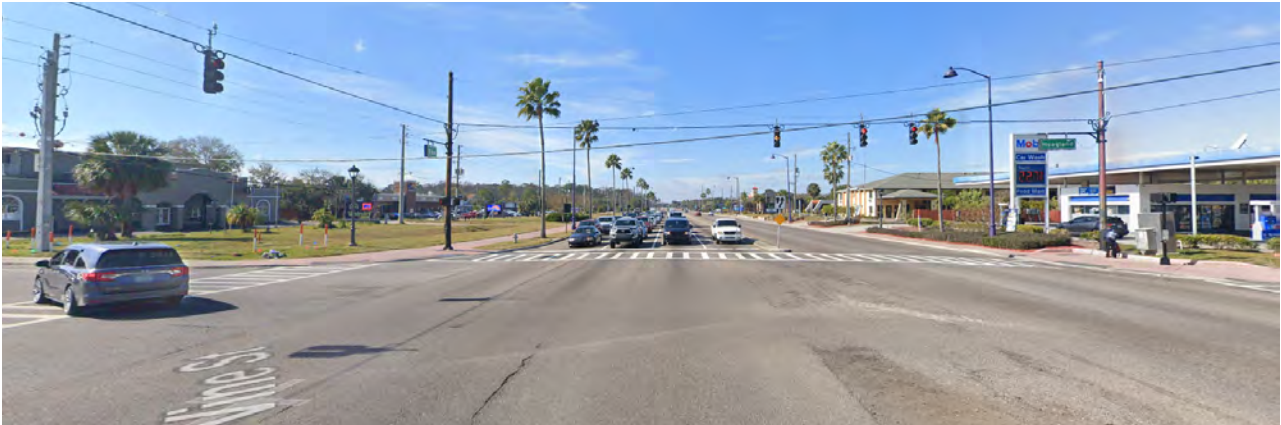
Looking west at Hoagland Blvd.
