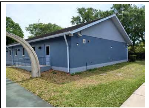
View at east end gable
