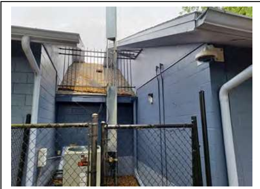
View at rear roof connector area
