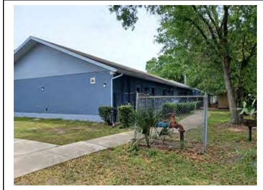
View at rear of building
