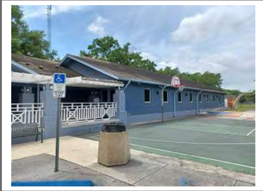
View at front of building
