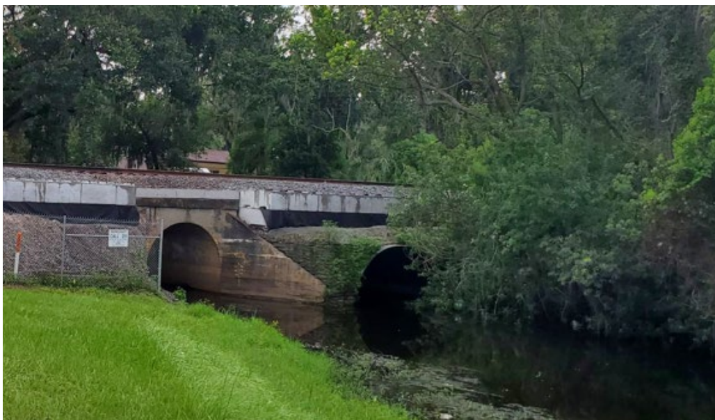
Figure 1 - Looking west at east side of culverts.
