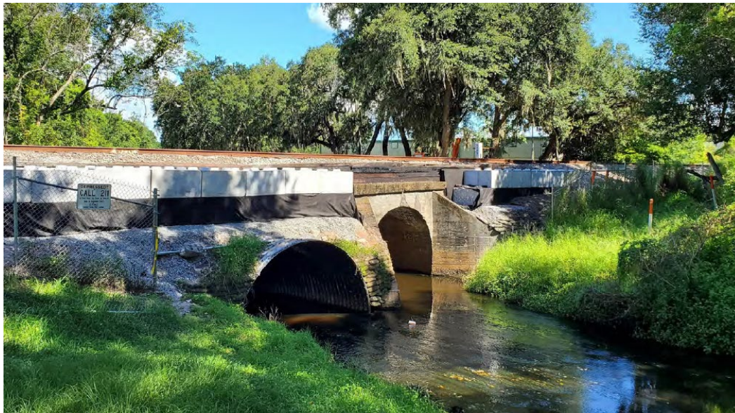
Figure 2 - Looking east at west end of the culverts.
