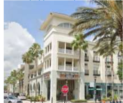
Figure 5 - 28: Small Footprint Tower (top) and Cupola (bottom)
