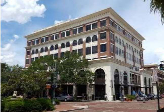
Office building with ground floor retail.
