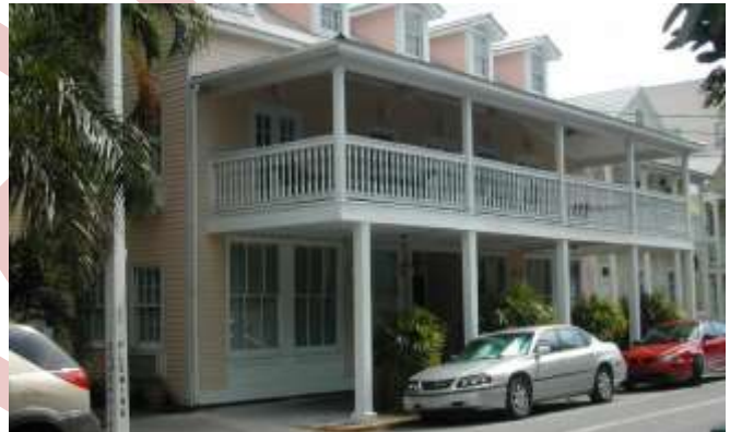
A two story wood framed gallery
