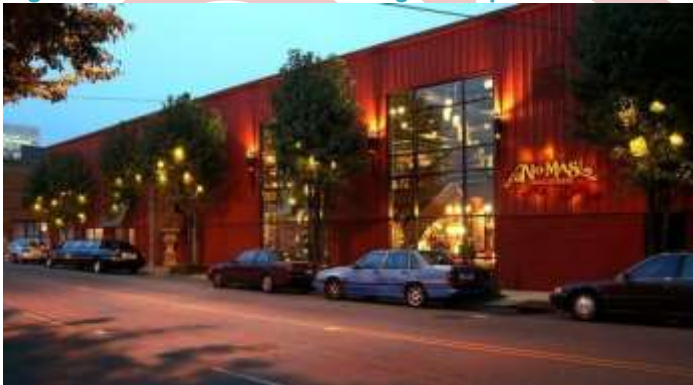
Figure 5 - 57: Industrial Building Examples
