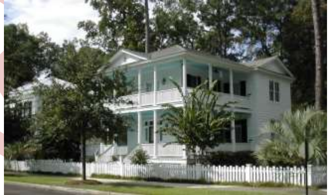
A 2-story porch on a single-family home
