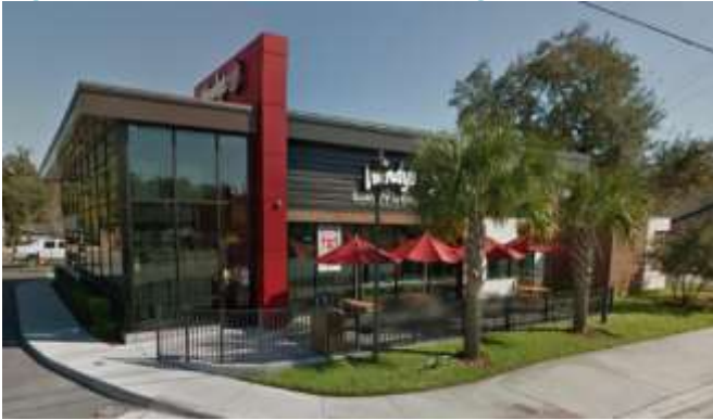
Figure 5 - 51: Exterior Drive-Through Facilities
