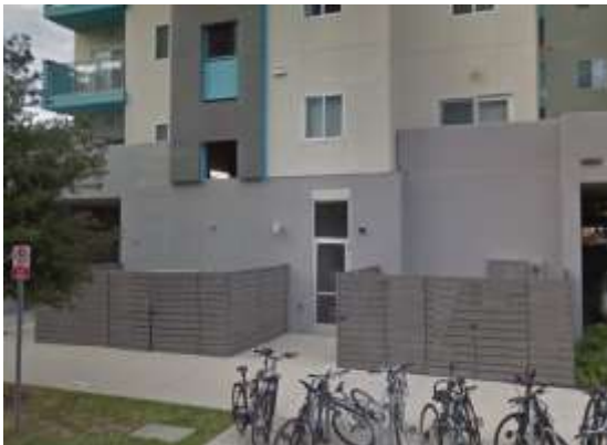
Allowed (utilities screened by fence)
