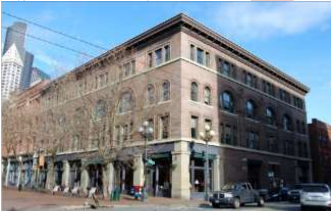
Taller ground to ceiling heights on the first floor provide flexibility for commercial use and a comfortable adjacent space for pedestrians
