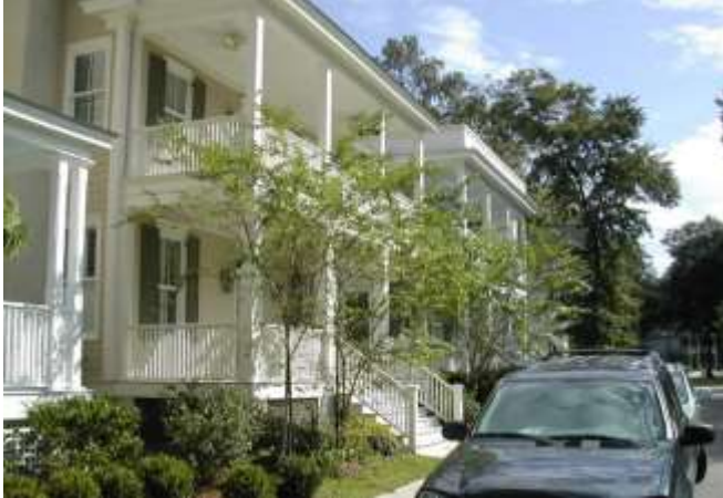
Closely spaced detached single family homes. A shallow front setback and strong cornice line create a more urbane streetscape
