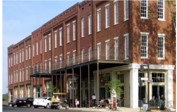
Mixed-use building with well-defined street edge. Horizontal articulation breaks the building into several distinct sections.
