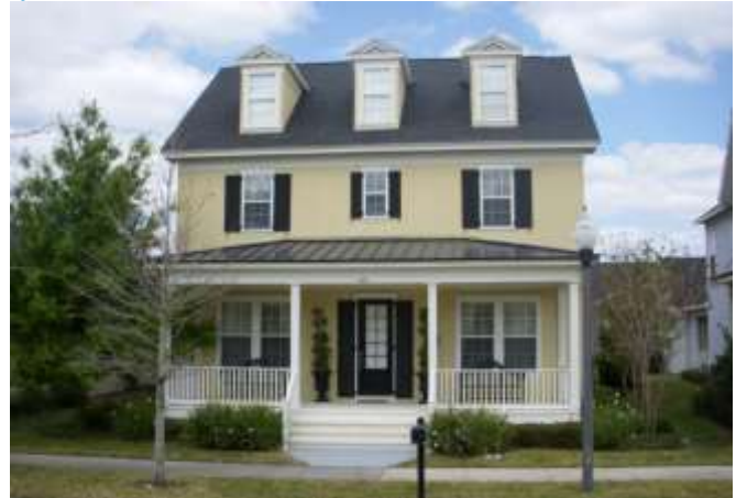
A two-story single family detached home with front porch
