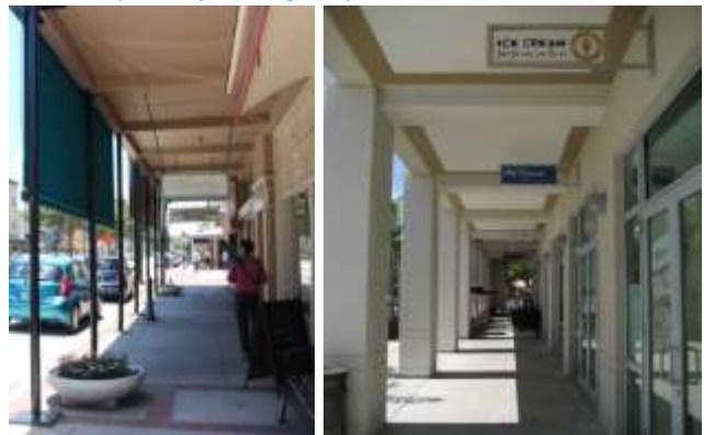
A gallery with slender metal columns (left) and masonry (right)
