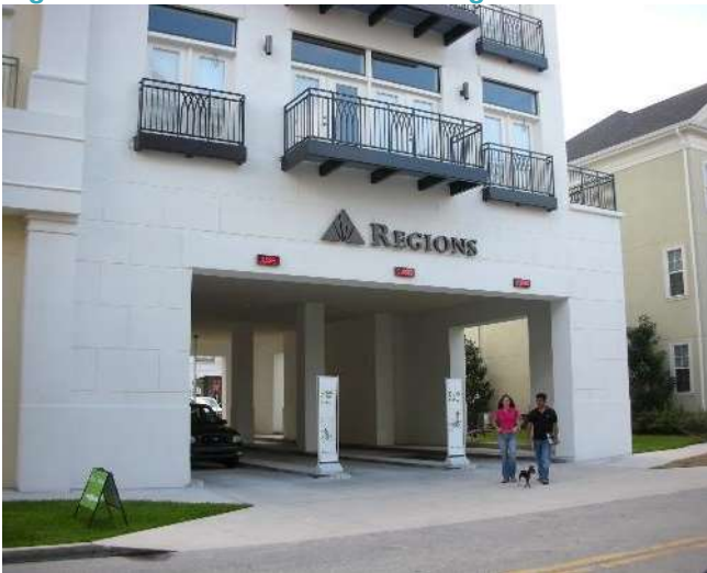
Figure 5 - 52: Interior Drive-Through Facilities
