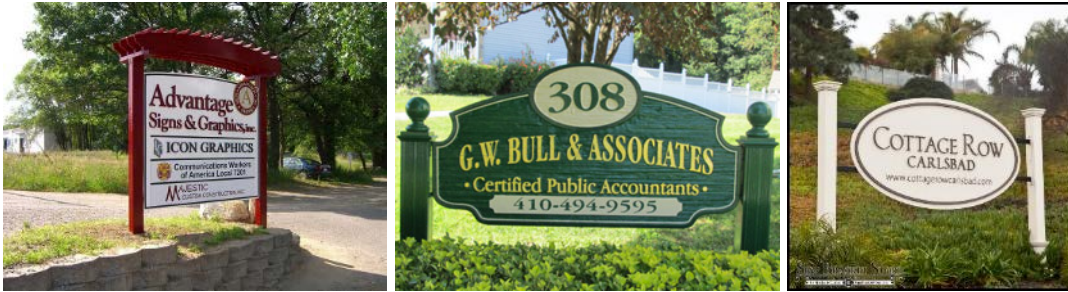
Figure 11- 19. Exposed Sign Structure
